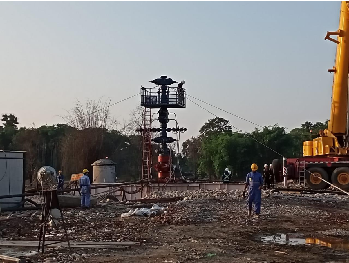
Pre-snubbing operation activities in progress at site, today
